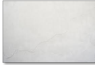
Hairline Cracks
