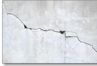
Structural Cracks
